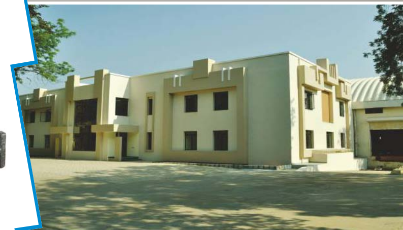
Photographs of a few Manufacturing Units
