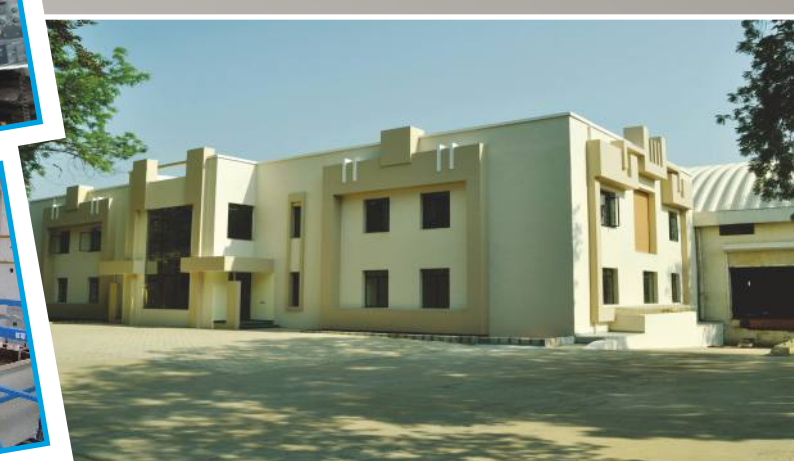
Photographs of a few Manufacturing Units
